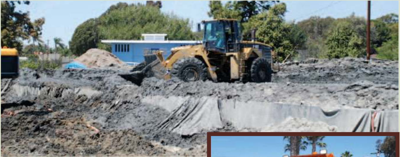
(Above Left) Cat wheel loader rented from Heavy Equipment Rentals moves and loads filtered silt, sand and dirt onto end-dumps for transport to the Port of Long Beach to be used as fill material. (Above Right) Sweeper rented from HER keeping dirt and dust levels down to a minimum.
