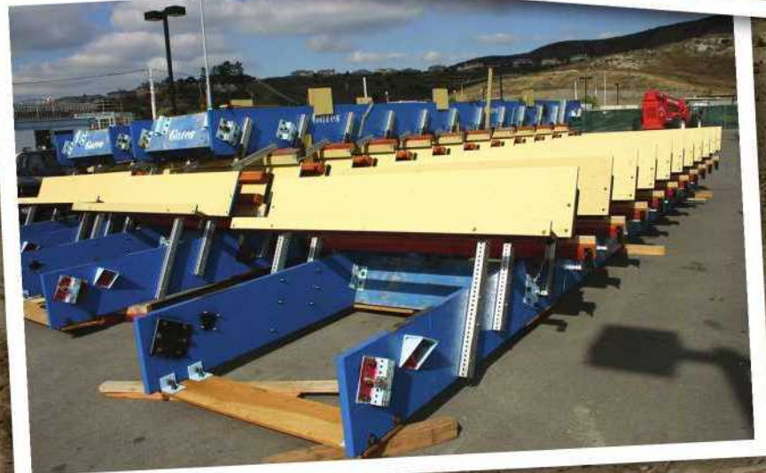
(Top Right) One of several excavators rented from Heavy Equipment Rentals, LLC. (Bottom Right) Some of the forms used in the construction of the concrete bleachers.
