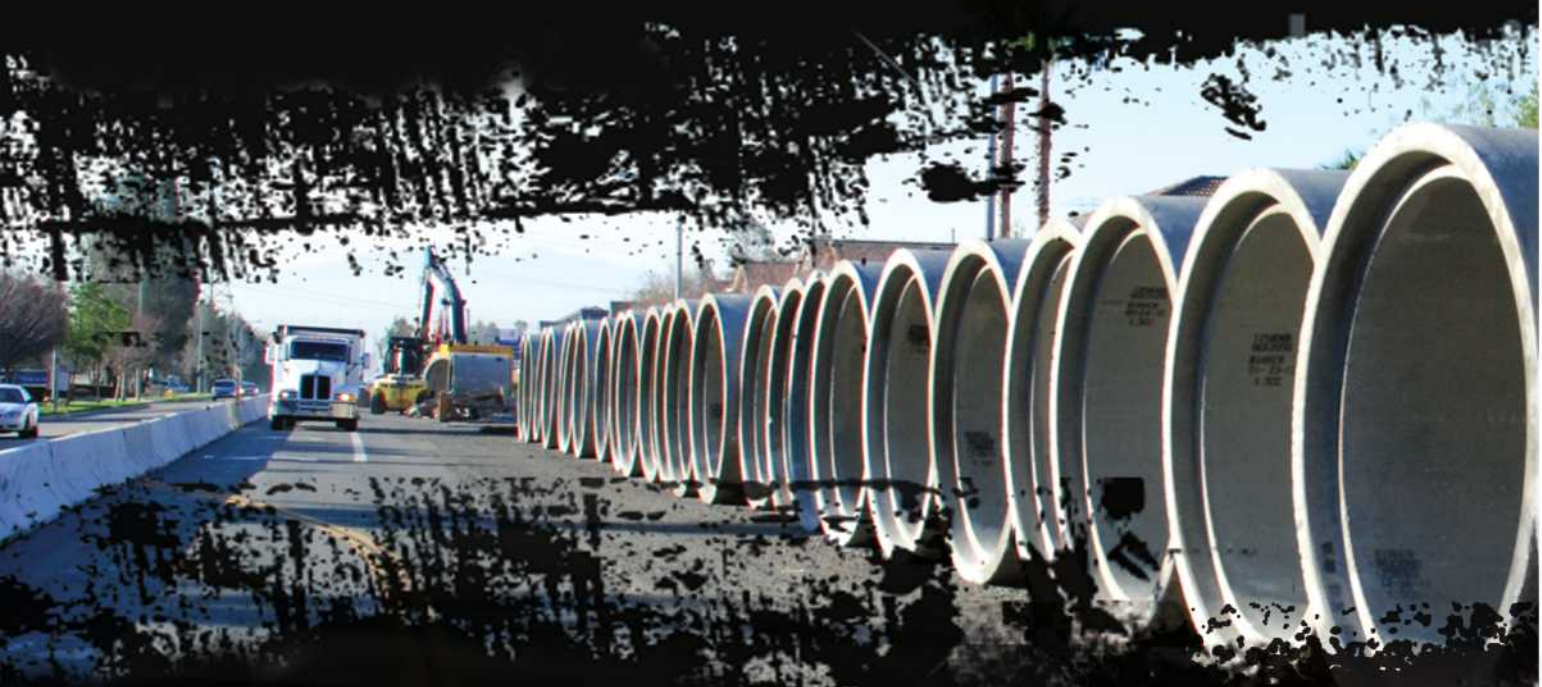
Sully-Miller Contracting knew they would need a very large excavator onsite to handle the installation of the 96" concrete storm drain.
