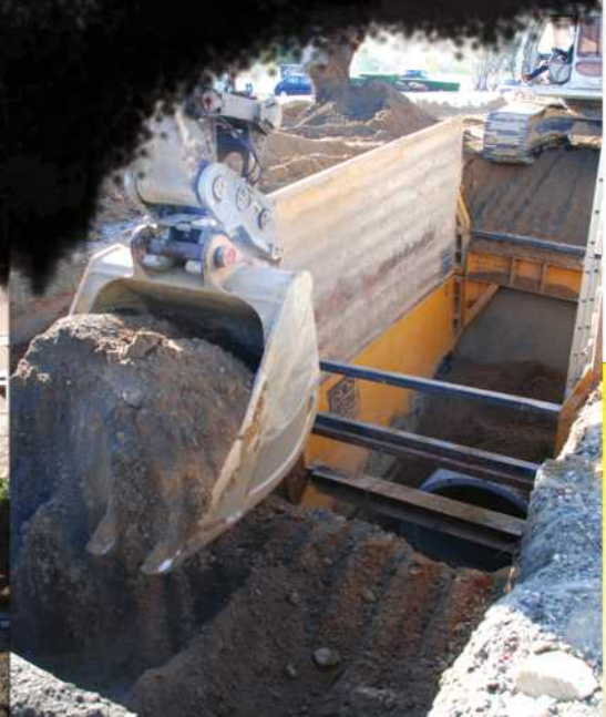
Sully-Miller Contracting knew they would need a very large excavator onsite to handle the installation of the 96" concrete storm drain.
