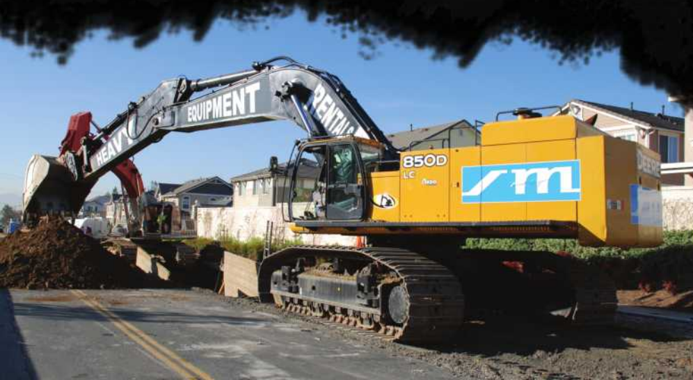
Sully-Miller Contracting knew they would need a very large excavator onsite to handle the installation of the 96" concrete storm drain.
